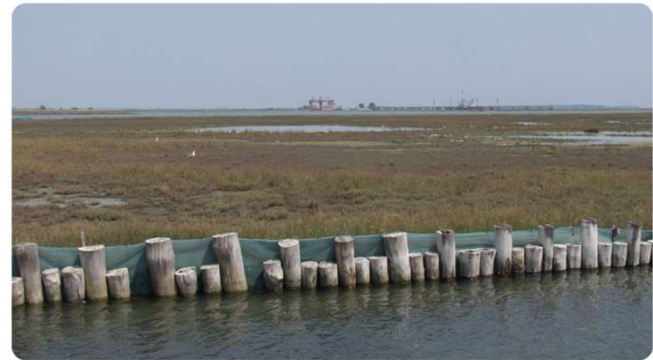
Piling technique to protect salt marsh edges
